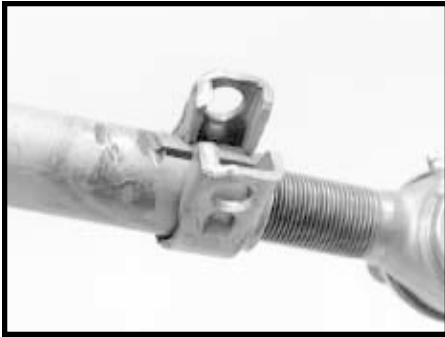
Cracks, breaks or bends
